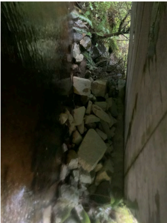
Left Bank Abutment when facing downstream
