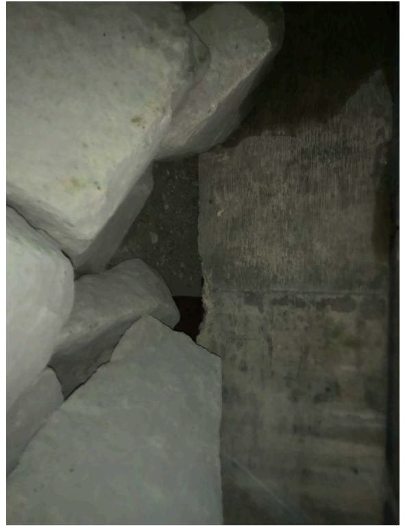
Right Bank Abutment when facing downstream
